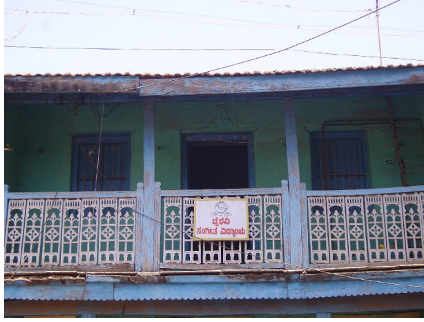
The Bhairavi School of Music Kannada building in Bailhongal
