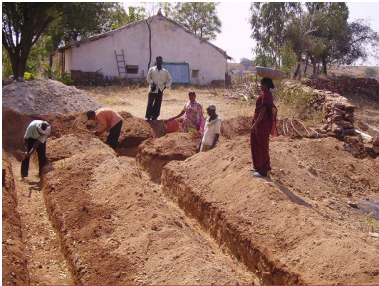
work at starting foundation level present building of Nadayoga Ashram
